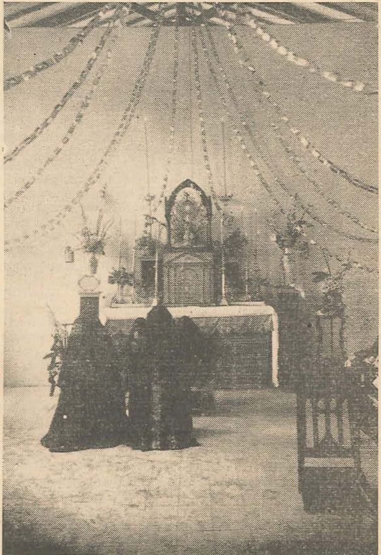
CAPILLA DEL HOSPITAL
